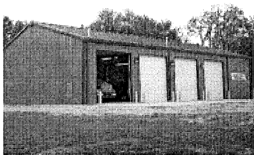
Linn County - Fire Station
