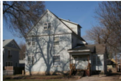
1031-1033 SW Western East elevation. 03/28/2013. KSHS.
