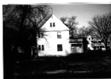
1031-1033 SW Western East elevation. n.d.
