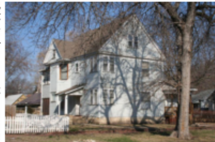
1031-1033 SW Western South and east elevations. 03/28/2013. KSHS.
