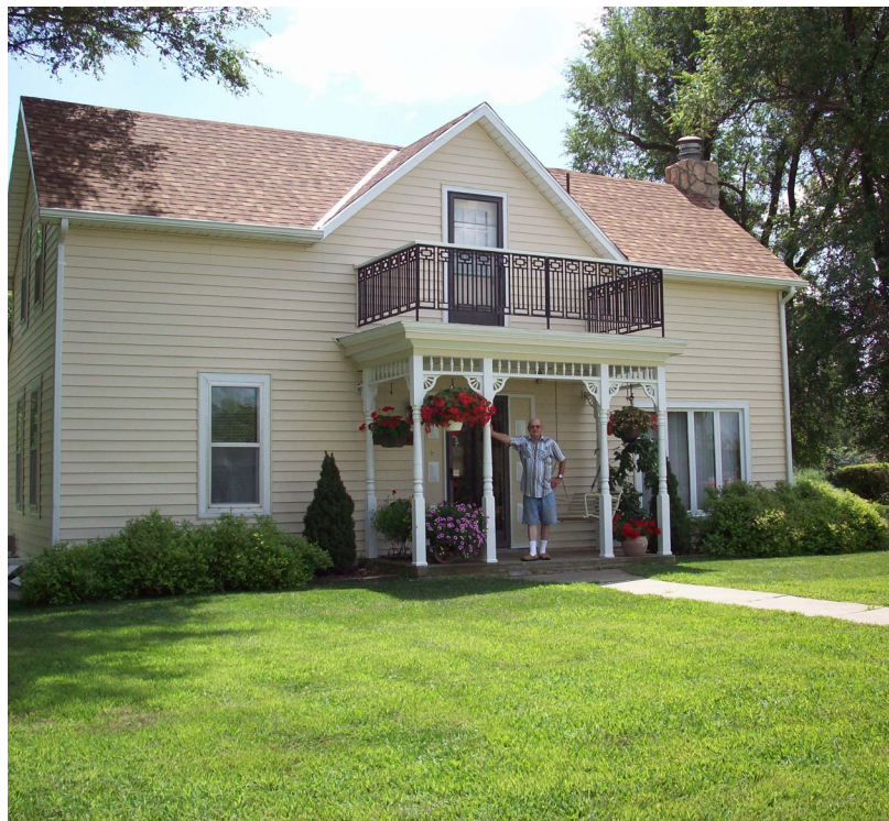
A single-home housing project in Linn County.
