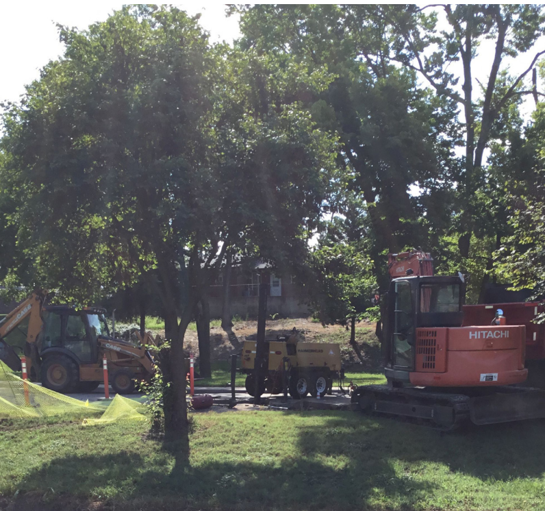
Wastewater improvement construction in Strong City.
