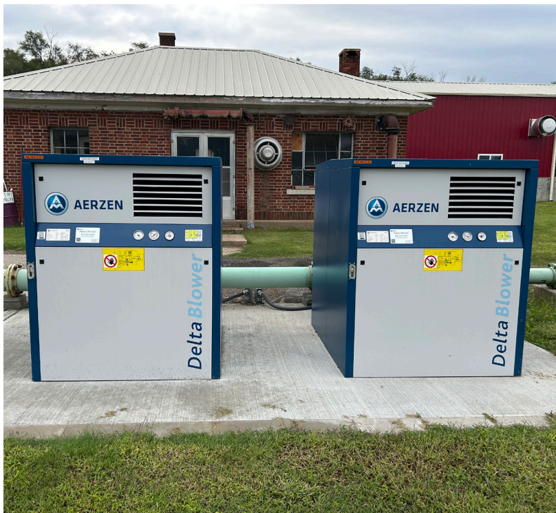
The city of Herington used an Urgent Need grant for the immediate replacement of failed aeration blowers at its wastewater treatment plant.
