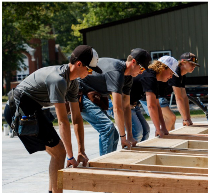
Labette County High School partnered with the city of Bartlett to build a house.
