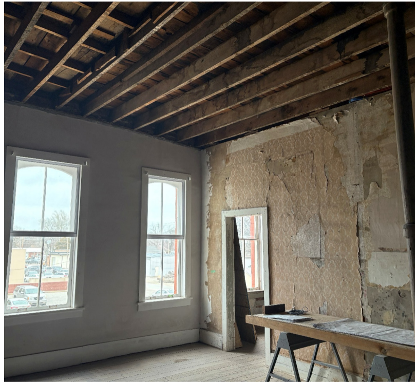
The historic Shay Building in Sterling is a ROOMS grant project. This project will offer four apartments in the downtown district once completed.
