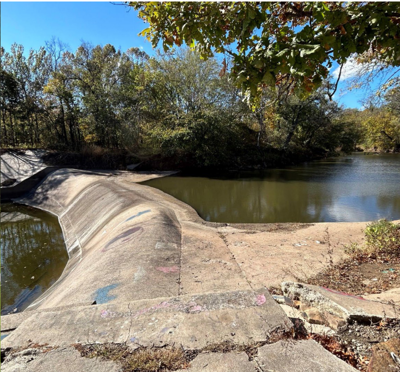
CDBG funding will be used to provide improved water access in Coffeyville and Caney caused by low water levels in the Little Caney River.
