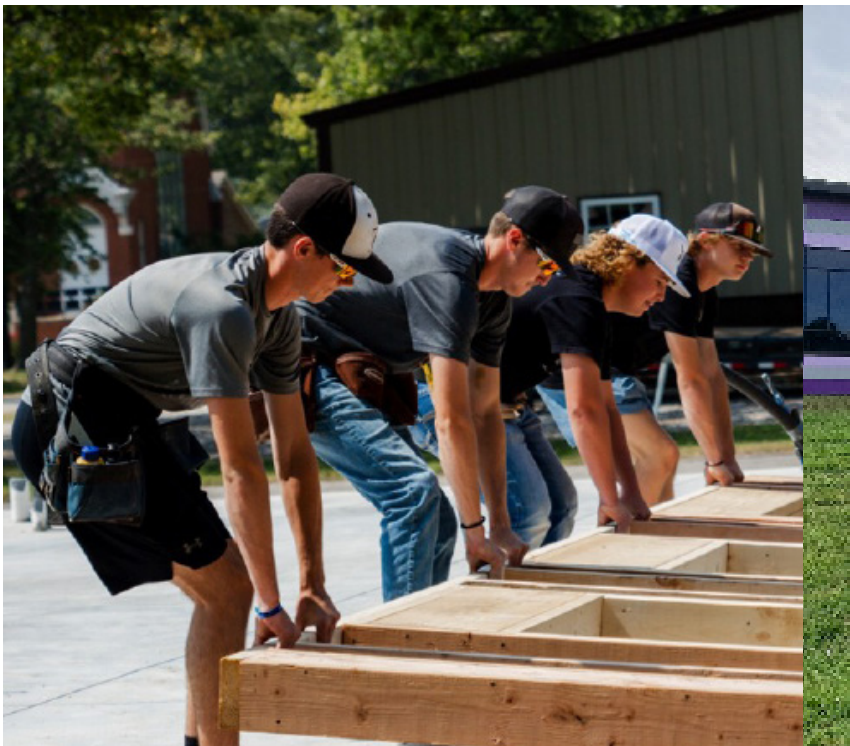
Labette County High School partnered with the city of Bartlett to build a house.
