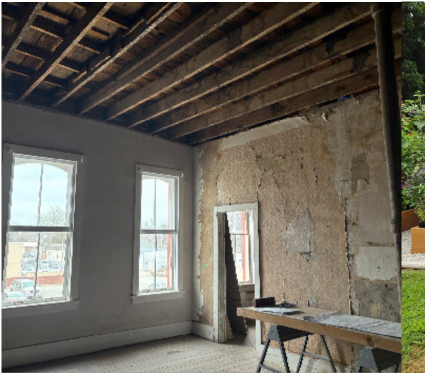
The historic Shay Building in Sterling is a ROOMS grant project. This project will offer four apartments in the downtown district once completed.
