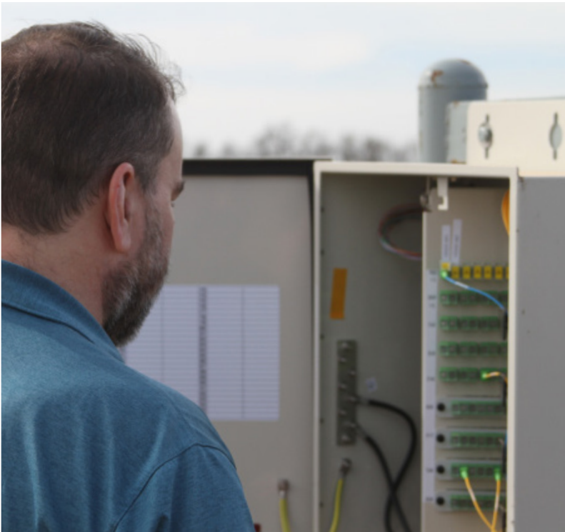
KOBD staff reviews broadband infrastructure during a site visit for a BAG 2.0 project in Harper County that was awarded to SC Telcom.
