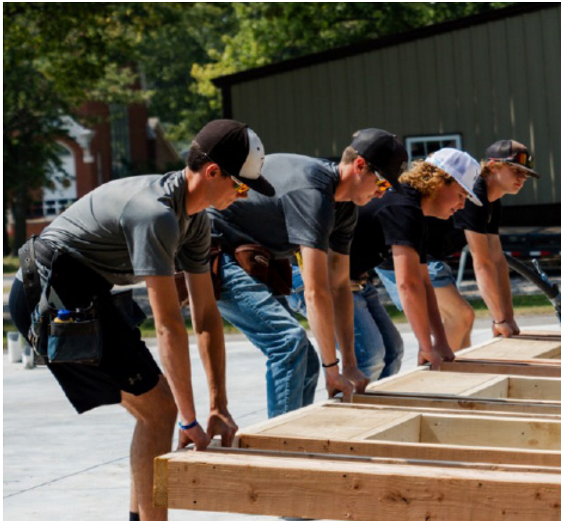
Labette County High School partnered with the city of Bartlett to build a house.
