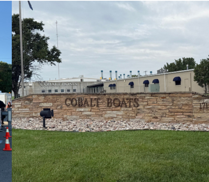
The city of Neodesha used Economic Development funds to repair street infrastructure necessary to retain jobs at Cobalt Boats.
